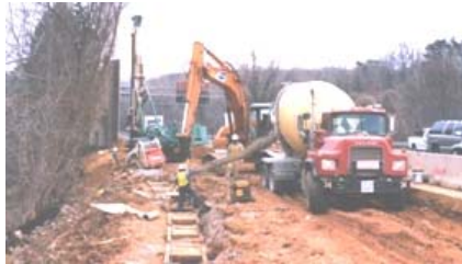
Drilled caissons averaging 20 feet deep are filled with concrete.
