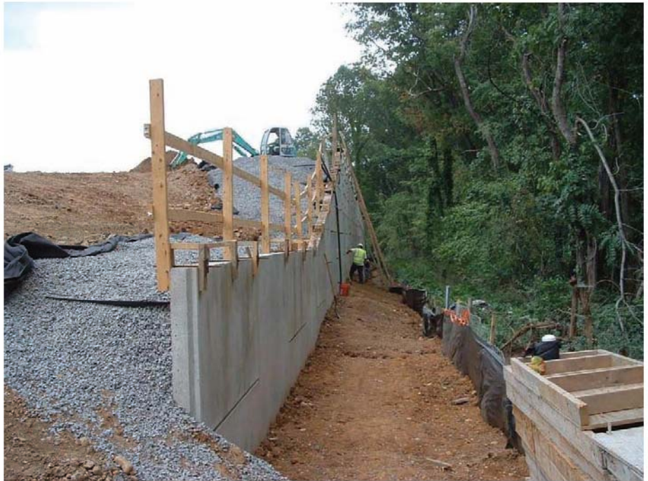
EarthTec Geostrap MSE Wall Holiday Inn Express Project, Alexandria, Va
