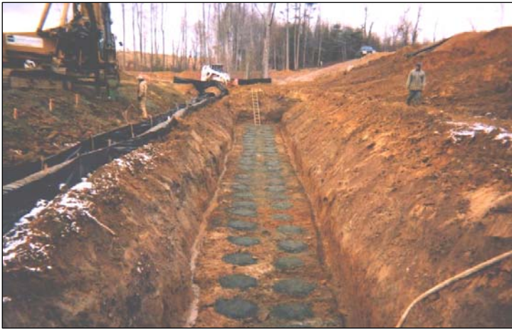
Geopier elements supporting structure
