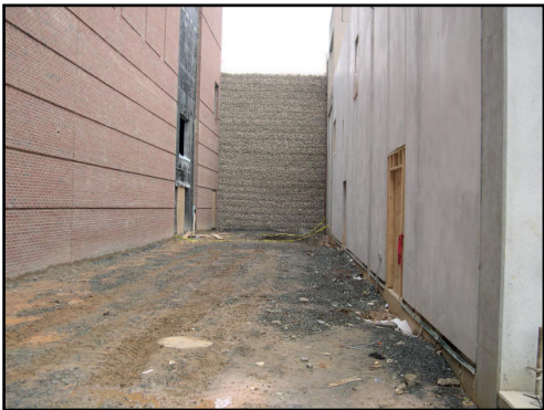
MSE wall at the Northwest corner of the Arena - March 25, 2005
