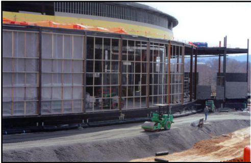
Main Entrance of the Arena with MSE Retaining Wall in the Foreground - March 10, 2005
