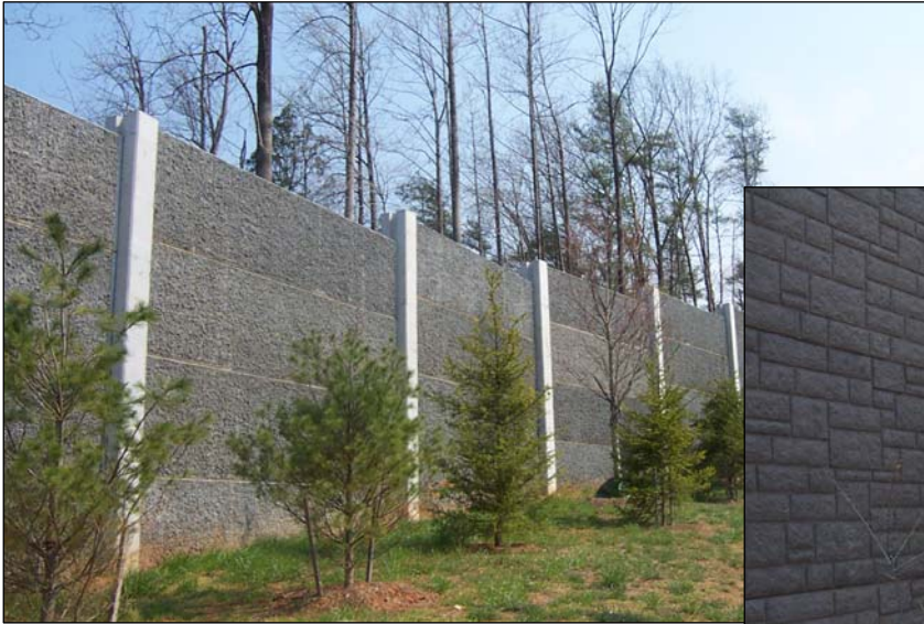
Concrete Posts with Reflective Concrete Fuzzy Rake Finish (Residential Side)
