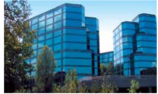
International Place Towers III Memphis, Tennessee
