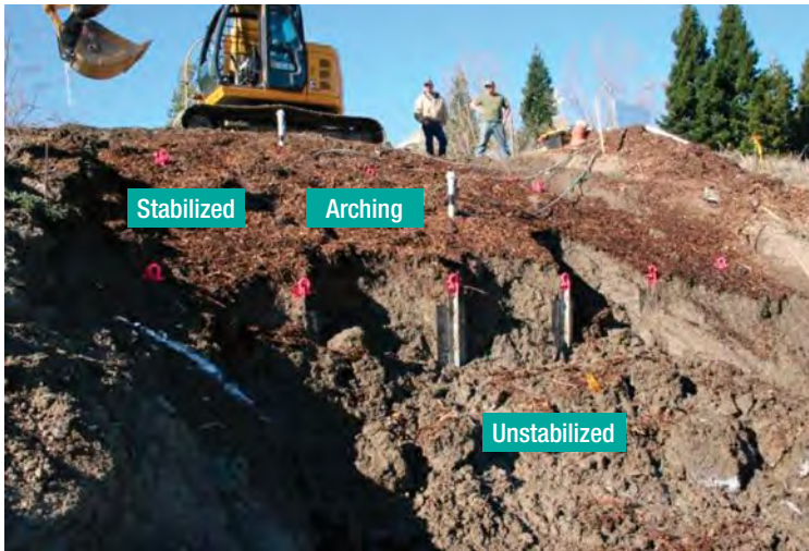
Figure 3: Plate Pile elements installed in full-scale test embankment.
