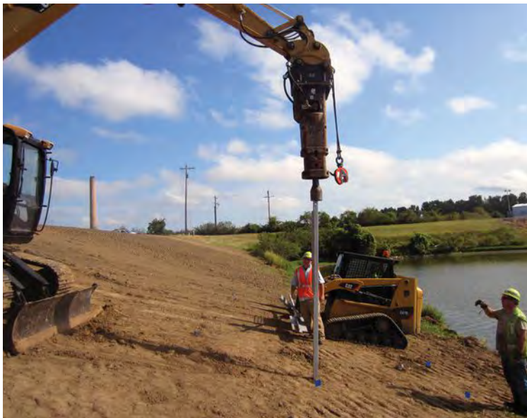
Figure 4: SRT system is installed to stabilize levees at an electricity plant.
