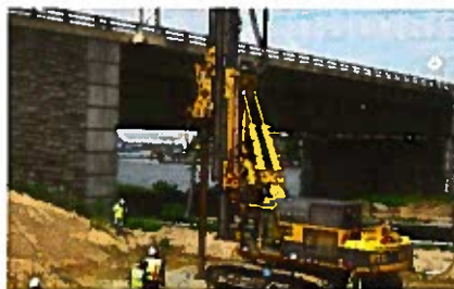
Installation of GCCs supports 35-ft-tall MSE abutment over compressible soils.
