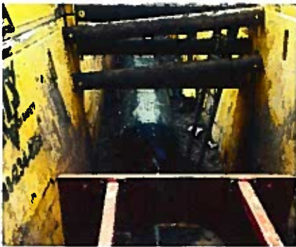
Swagelining a new Texas water main
