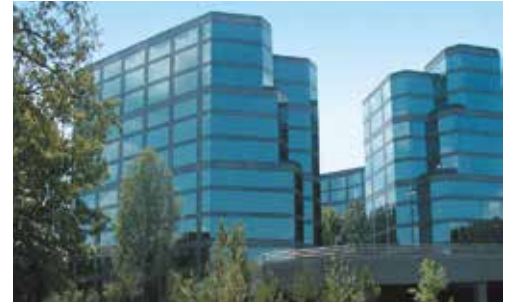
International Place Towers III Memphis, Tennessee
