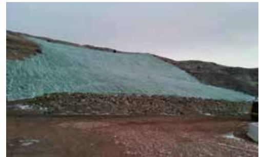
Carus Well Pad Slope Stabilization Near Killdeer, North Dakota
